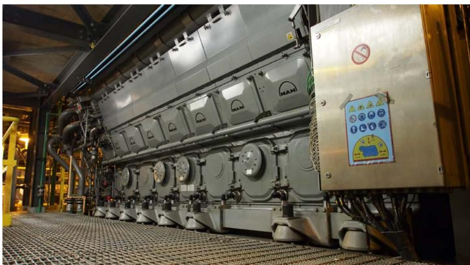
*Three engines of the type MAN 14 V32/40 CD provide electricity for the processes in the refinery.*
